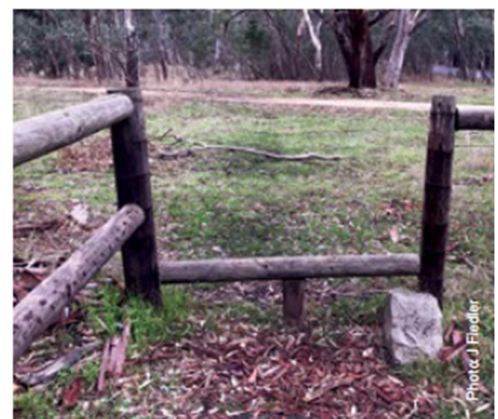
Step-over (1 rail) of timber with an informal 'ramp' stone to assist cyclists. Kuitpo Forest, South Australia. Photo: J Fiedler
