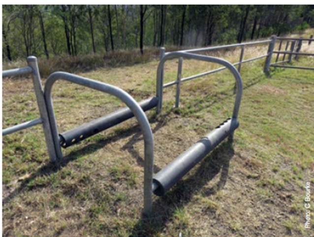
Step-over (2 rails) of metal with rubber sleeves to reduce noise, South-East Queensland.
