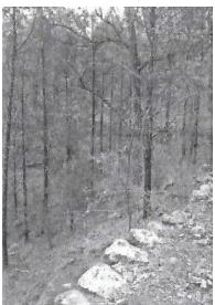
The **photograph at rig**ht shows the clever workmanship on an incline - the rocks at the edge of the track act as a bulwark, banking the road and protecting it from
